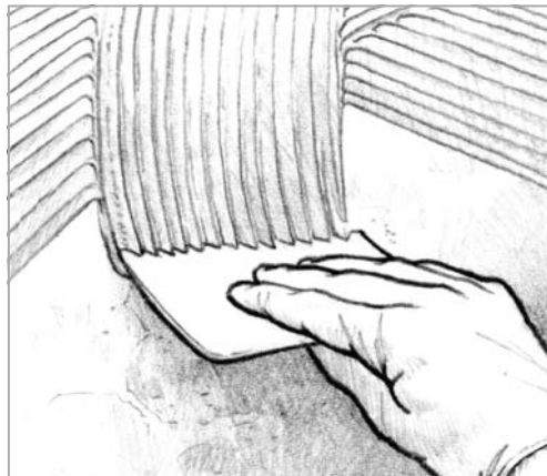
Figure 7 Apply the fairing compound with the notched spreader. Control the height of the ridges by the angle you hold the spreader.
